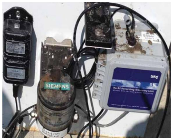
Figure A: Wireless Cellular Modem Sends Flow Data
